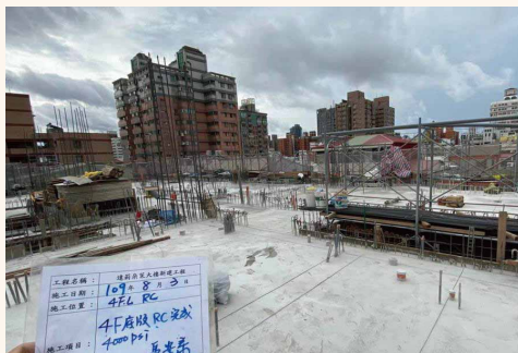
3F柱牆、4FL樑版混凝土澆置完成(8/3)
