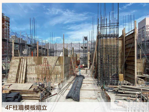
4F柱牆鋼筋綁紮
