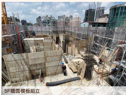
5F柱牆鋼筋綁紮
